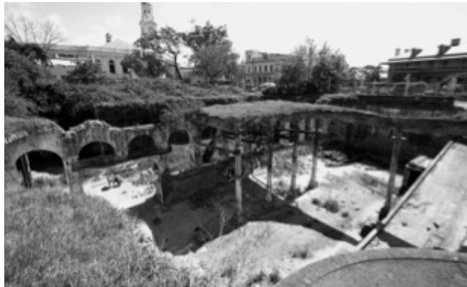
Western chamber, Paddington Reservoir, 2007, Photograph: Nathaneal Hughes.
