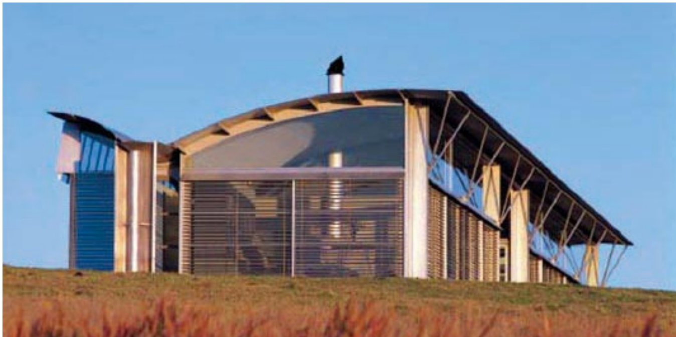
Magney House (Bingie Farm) , Glenn Murcutt, 1984 Moruya NSW. Creative Commons.
