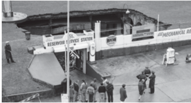
Collapse of part of the reservoir roof, Robert Pearce, Photograph: Fairfaxphotos, The Sydney Morning Herald, 1 July 1990.
