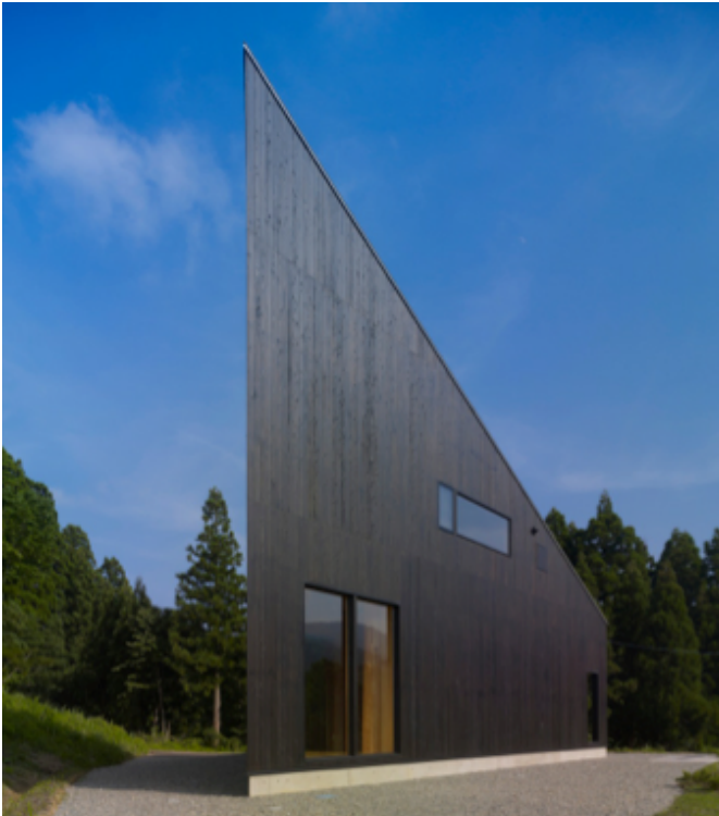
Australia House , West elevation highlighting the sharp edges of the triangular building and the steep pitch of the roof accentuating the geometrical form. Photography by Brett Boardman.
